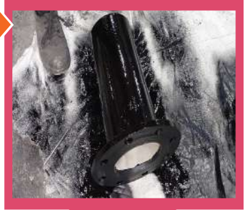
BITUMEN COATING
